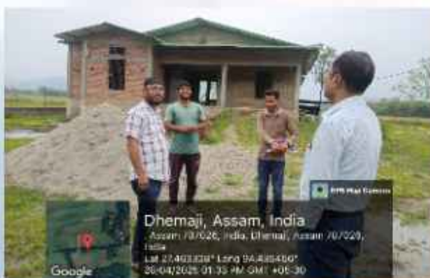
Working shed construction, in progress
